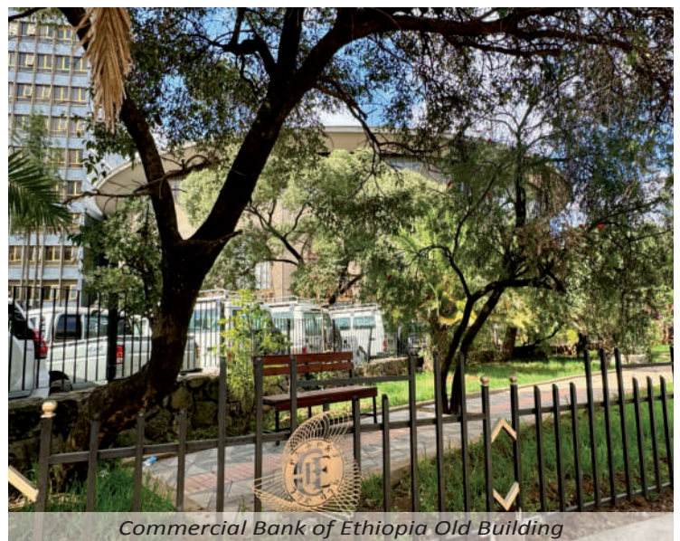
Commercial Bank of Ethiopia Tower Addis Ababa
